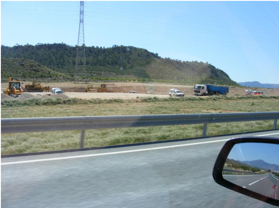
Construction work on the new motorway
