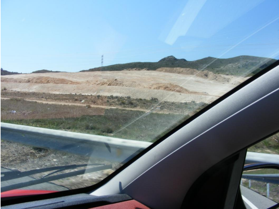
Motorway work close to SADM
