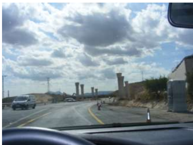
Motorway flyover works near Pinoso turn off
